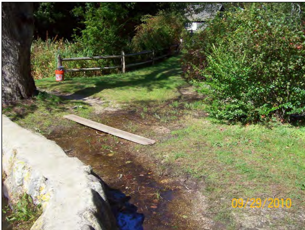
Photo No. 4 – Embankment crest viewed from spillway
