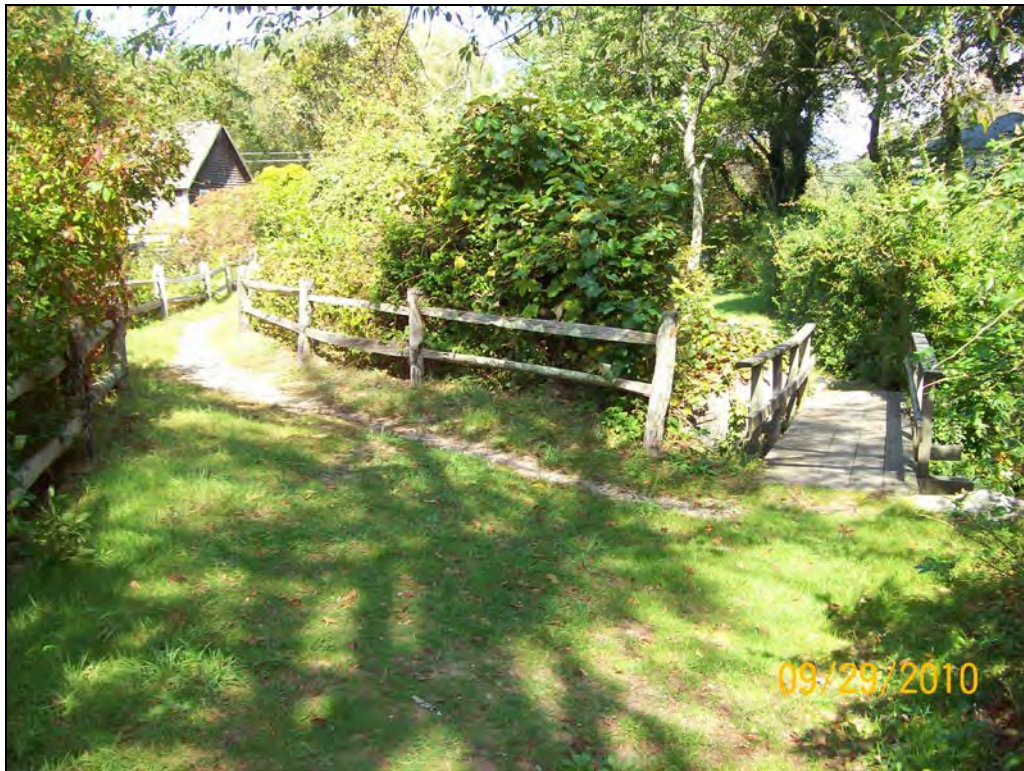
Photo No. 7 – Downstream side of embankment and transition to natural ground
