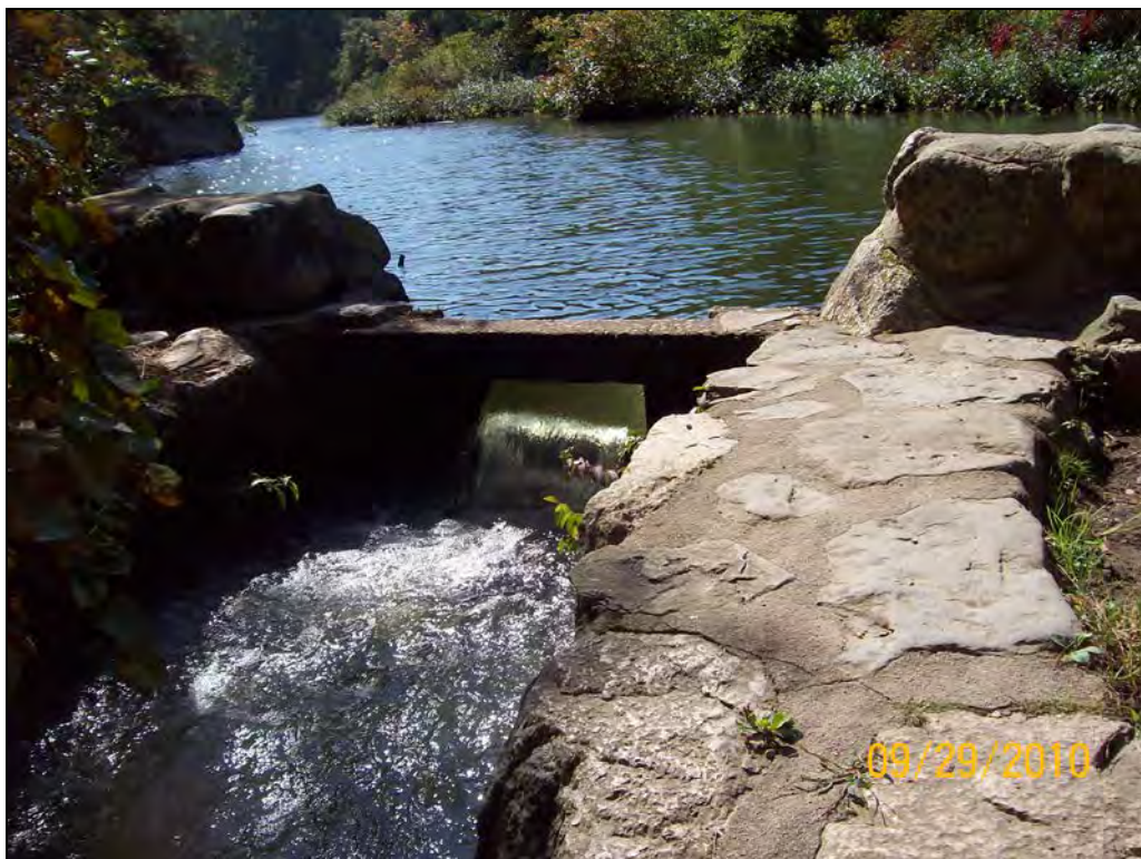
Photo No. 2 – Concrete spillway weir with rectangular orifice for fish passage
